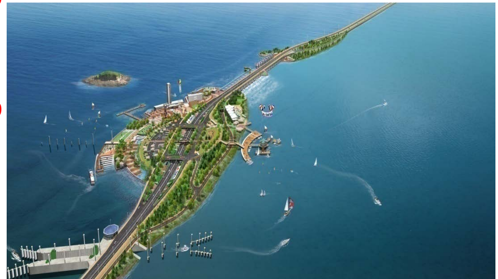
Sihwa, South Korea tidal power plant 2011
